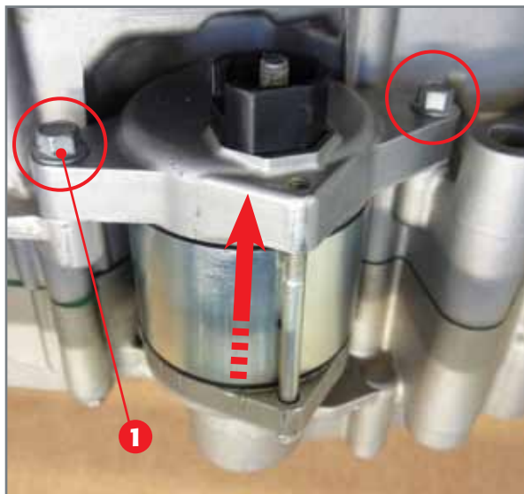
Removal of start motor.
